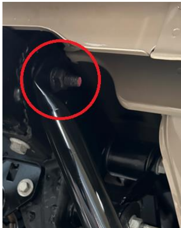
Photo 24: Pencil brace installation
